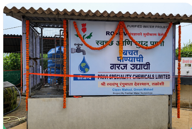
RO systems and water scheme upkeep, Mahad
