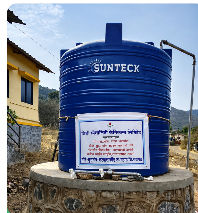
Kusgaon Kharbachakond water supply repair
