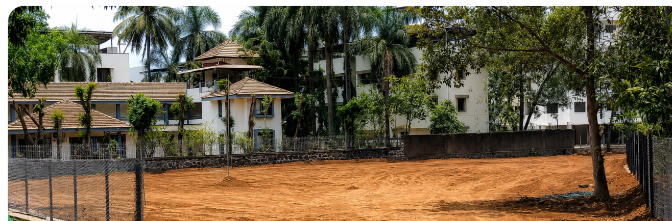
Construction of a joggers park
