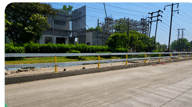
Safety crash guard installation, MIDC road
